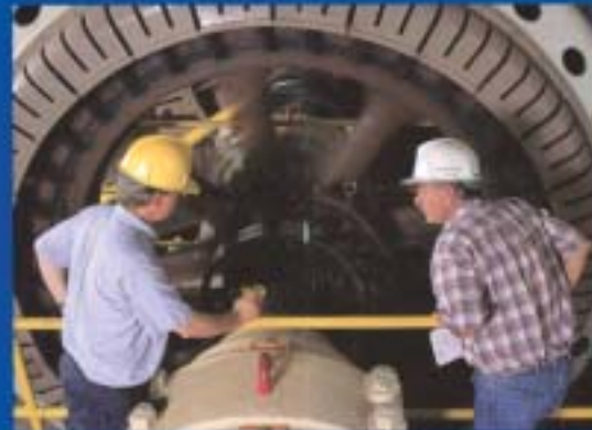
Morgan Falls employees regularly inspect the condition of the generators.
