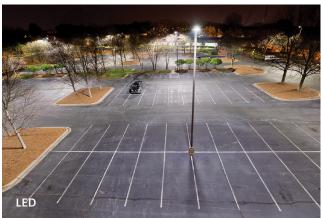
182 GE Evolve 202-watt Modular LED area fixtures. All fixtures have a Correlated Color Temperature (CCT) of 4000K and a Color Rendering Index (CRI) of 70. All existing poles and pole locations were used.
