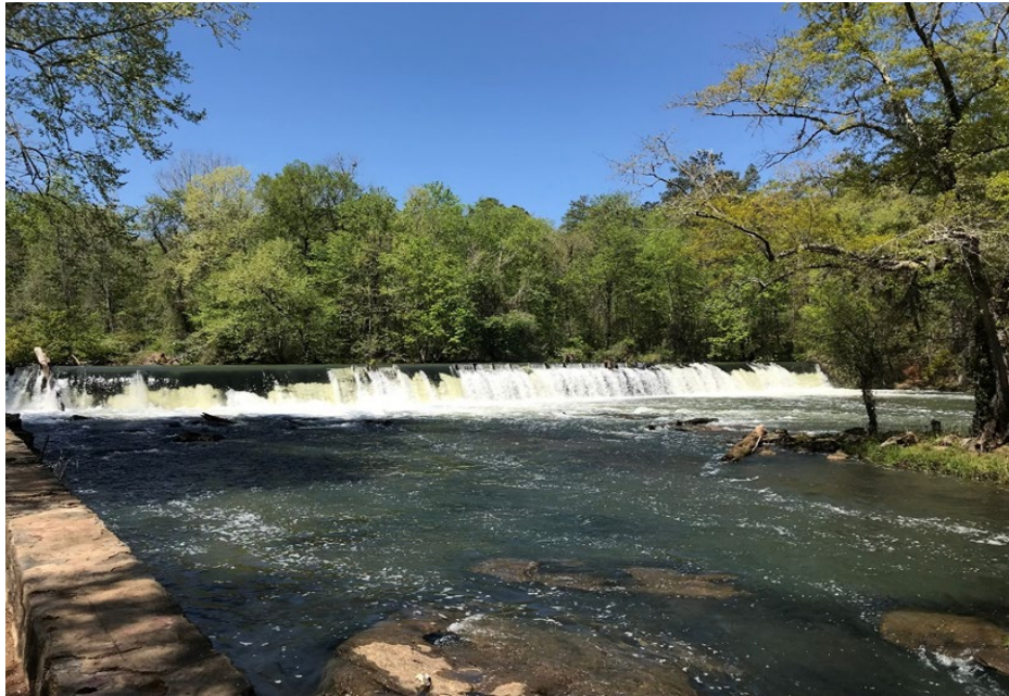
Source: Georgia Power 2018b
