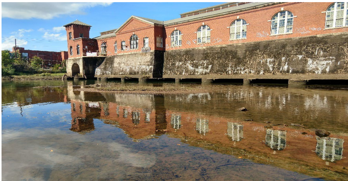
Note: View looking west from Georgia side at the Langdale Dam
