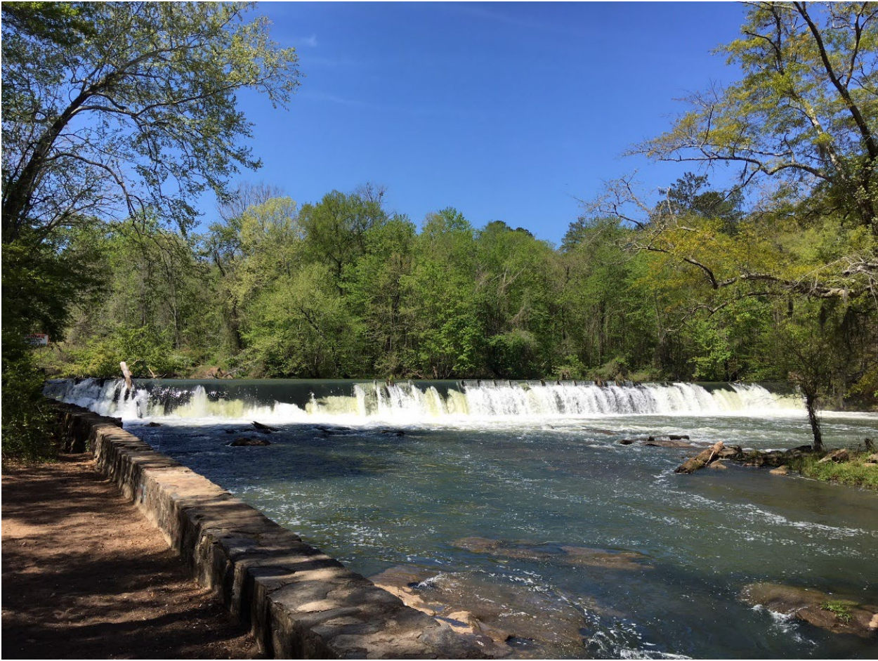
Note: View is standing on the mid-channel island downstream of the dam, looking upstream and north.
