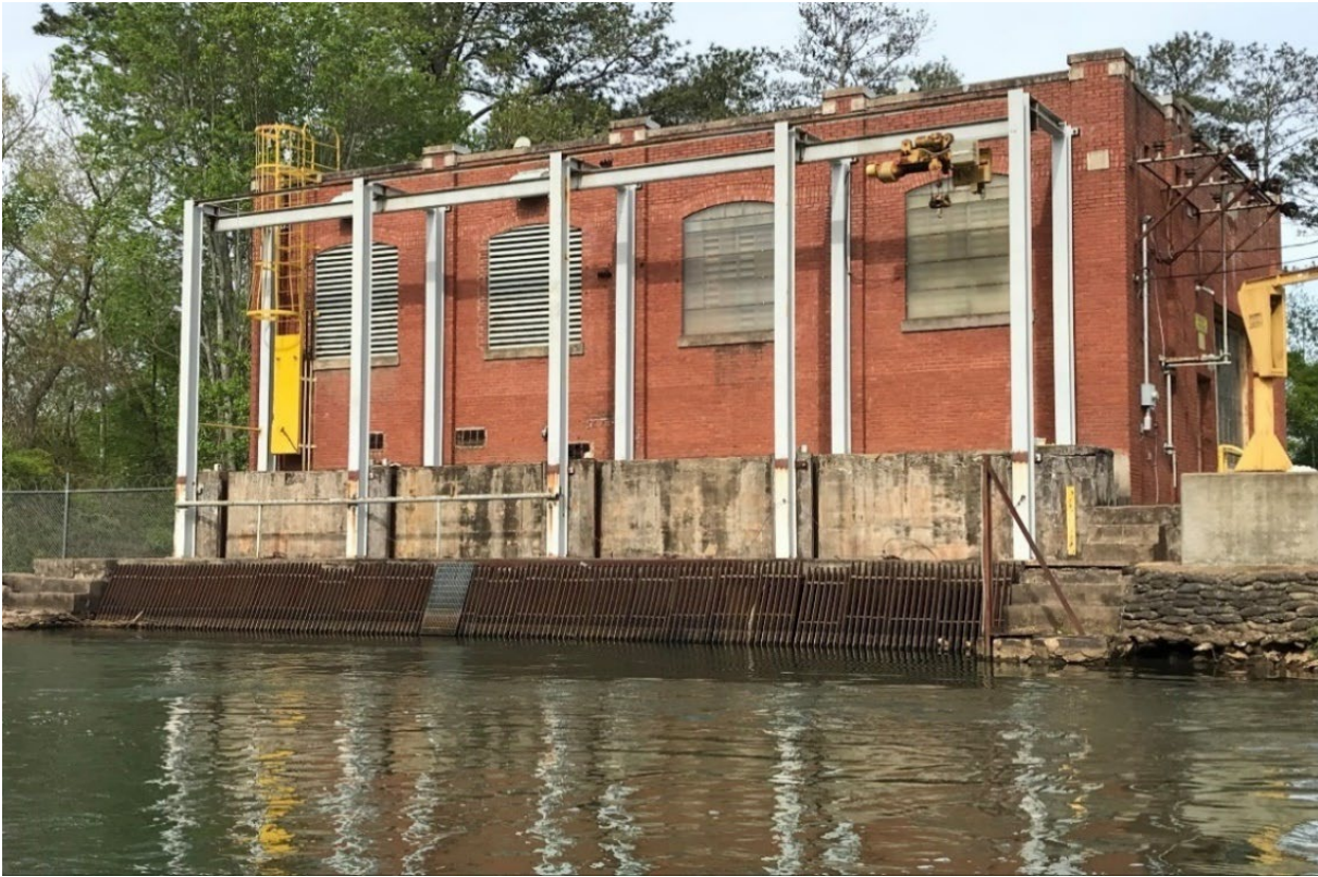
Note: View: from Riverview headrace channel above dam, looking downstream
