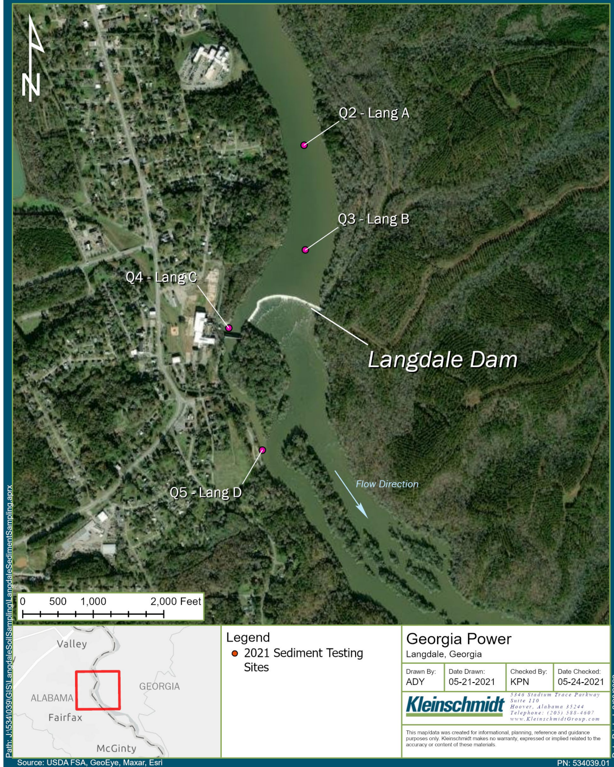
Figure 3-2 Langdale Sediment Testing Sites
