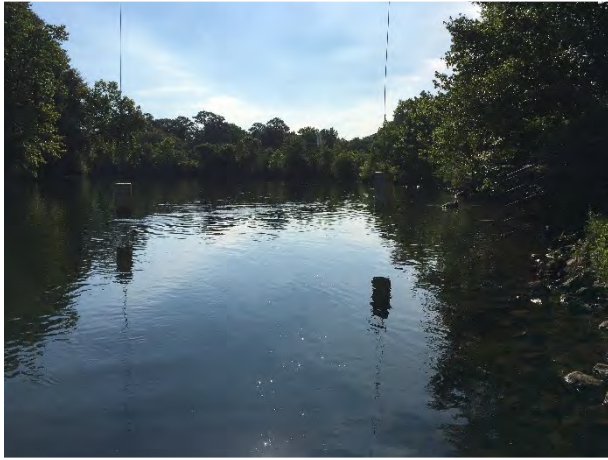
Photograph 1 - Western shoreline, upstream of dam.
