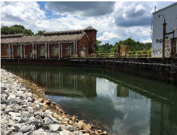
Photograph 3 - Langdale Dam generation facility.
