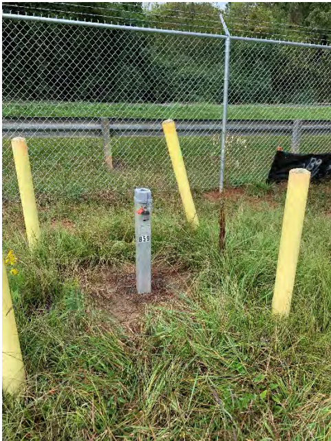
B-59 – Straighten bollard and clear overgrowth
