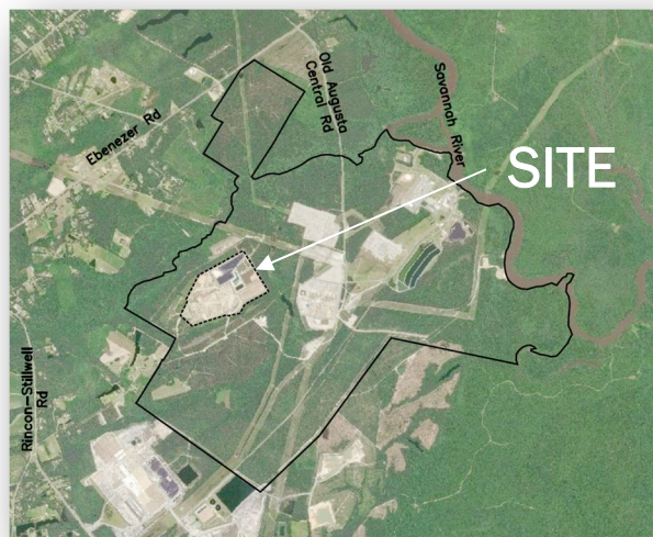
PLANT MCINTOSH AND SITE
