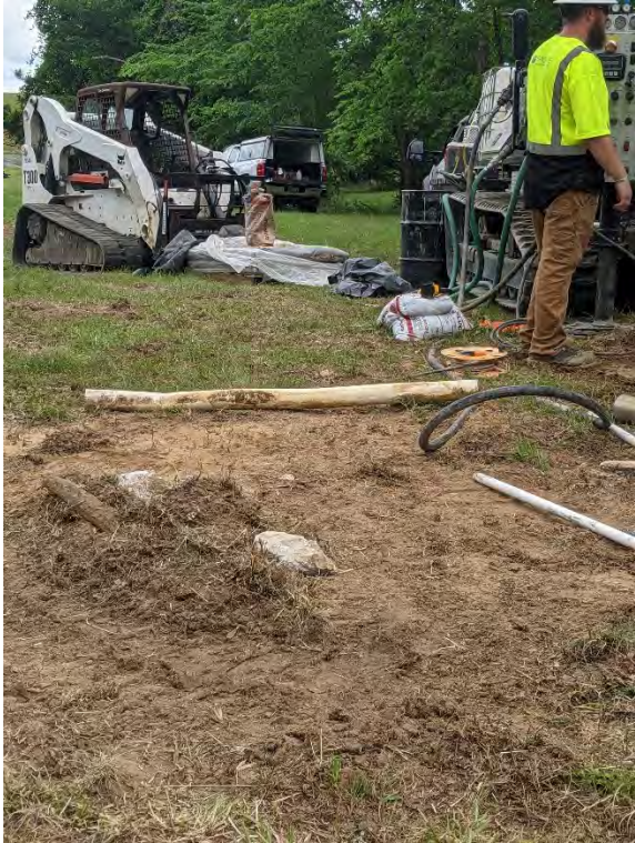
Well screen removed from bottom of well.
