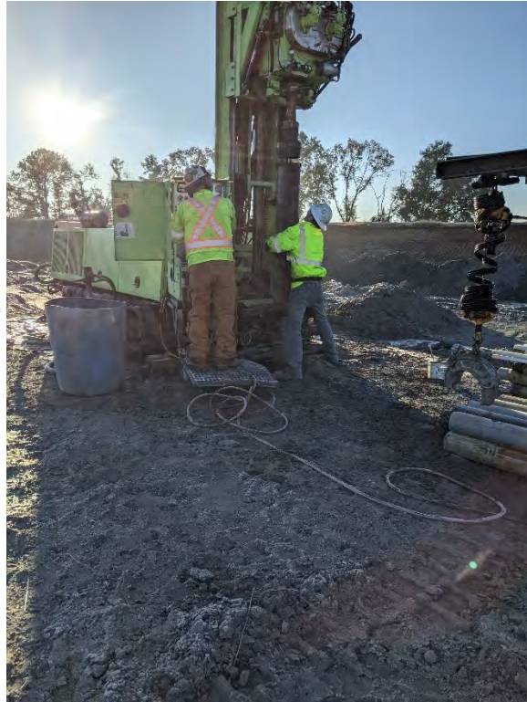
Overdrilling outer casing with 9-inch augers in upper 25 ft of the well down to bottom of ash pond.
