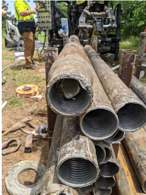
Part of casing inside auger.
