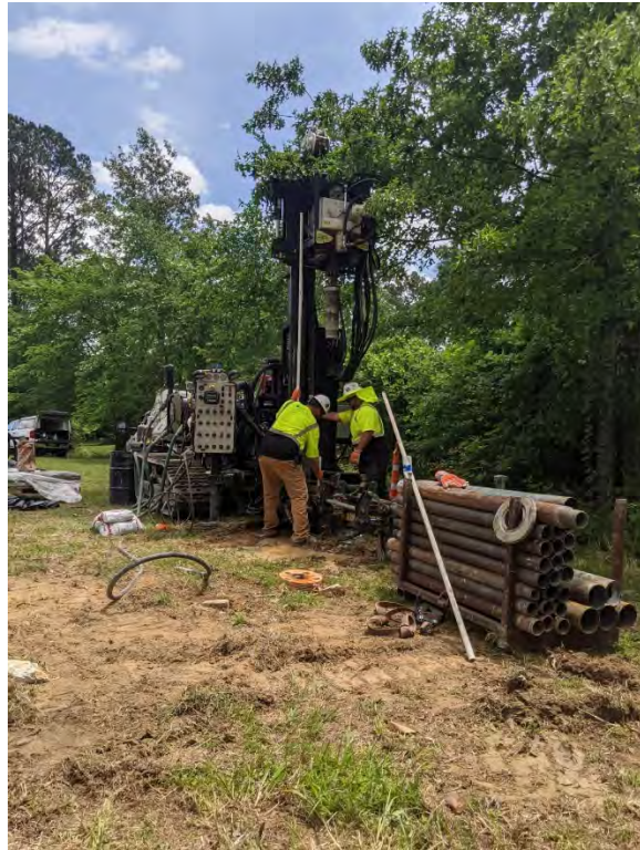
Two-inch inner casing of well overdrilled with 6-inch auger.
