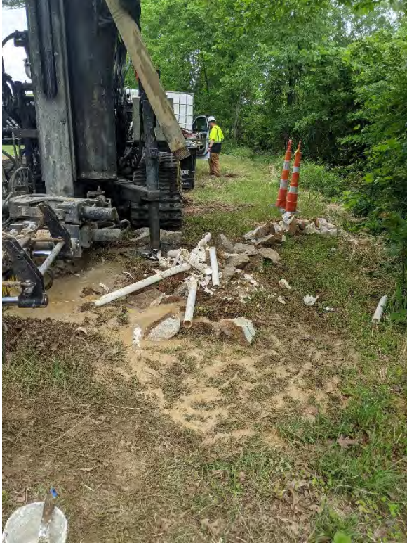
Complete well casing removed from well.
