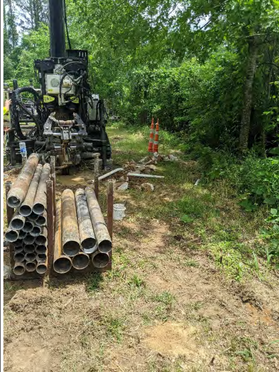
Removing part of well casing.
