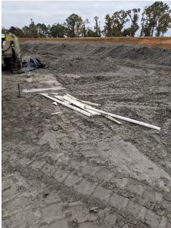
PVC pipe removed from well.
