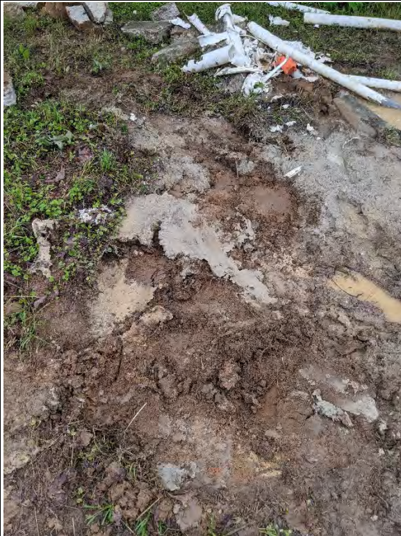
Overdrilled well grouted up to ground surface.
