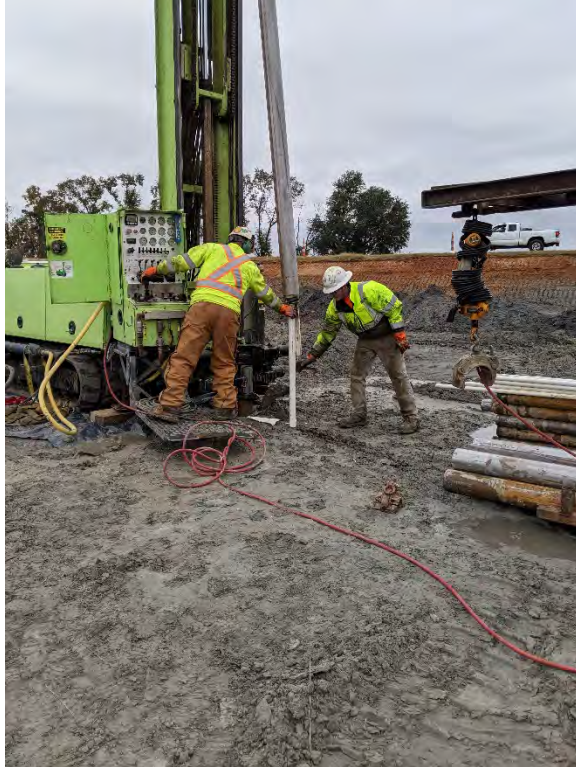
Removing final auger and 2-inch casing from overdrilled well.
