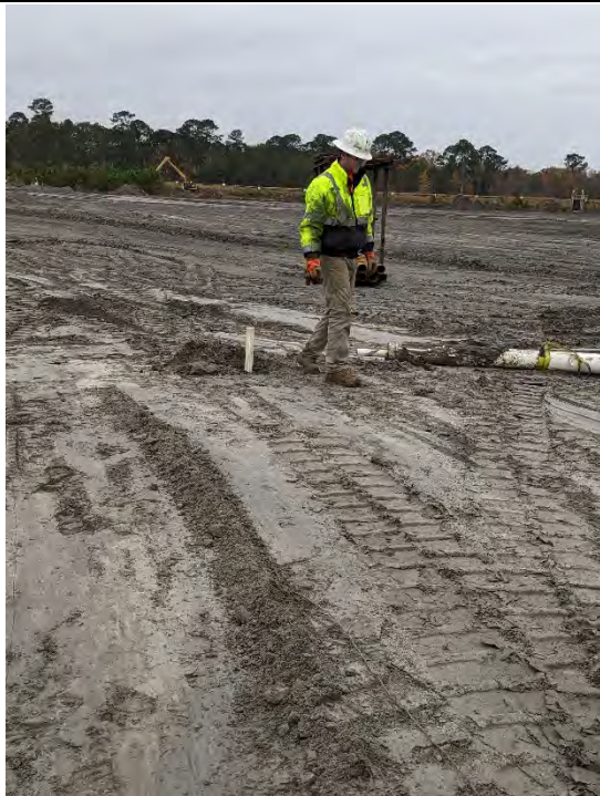
Casing above ground surface has been removed.
