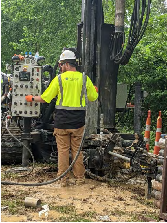
Grouting up borehole with tremie pipe.
