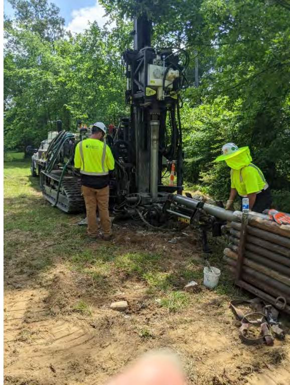
Begin overdrilling well to abandon well.
