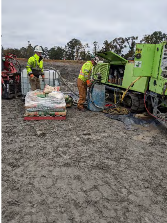
Mixing grout to backfill borehole to bottom of ash pond. Approximately 26.5 gallons
