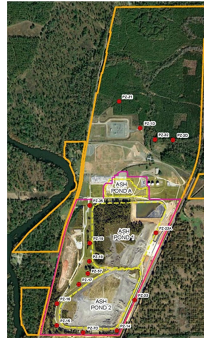
Plant Mitchell Ash Ponds A, 1, and 2
