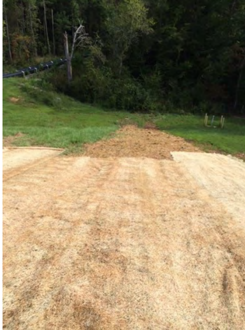
Exhibit 3 Embankment Repair Uphill from GWC-14.
