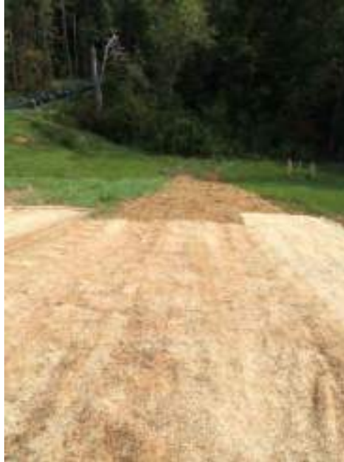
Exhibit 3 Embankment Repair Uphill from GWC-14.
