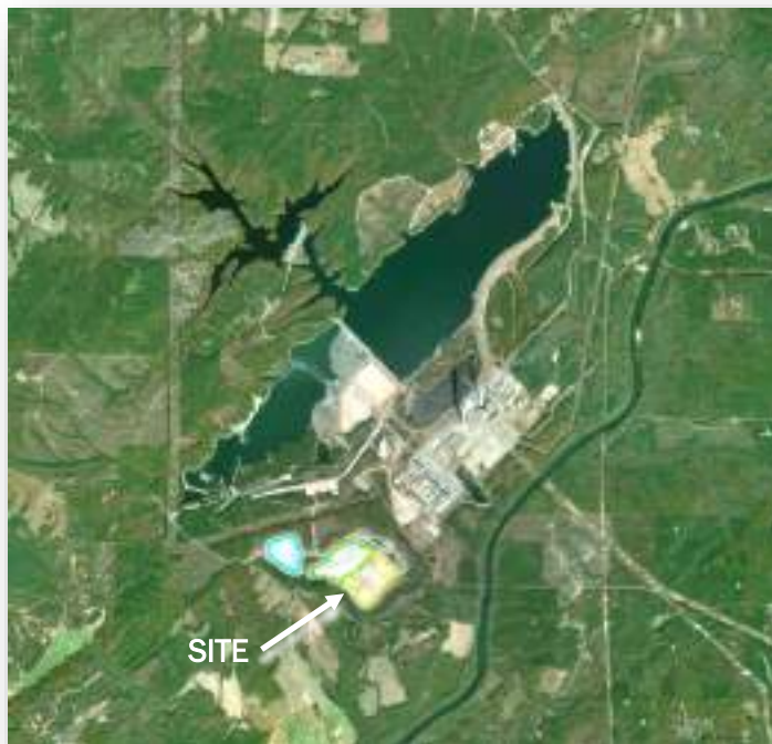
Plant Wansley and Plant Wansley Landfill
