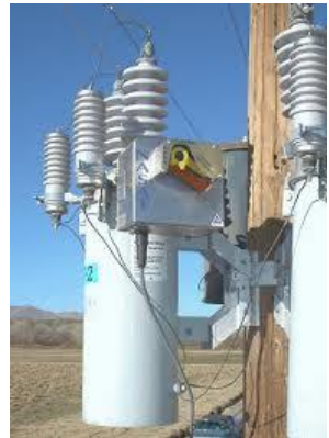
Hydraulic recloser – single phase application
